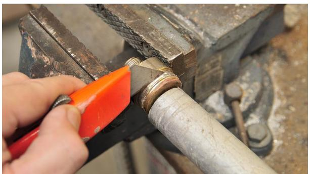
Above: Use a Stanley knife to get out the adhesive gunk from between the thread. Then, using an electrical contact cleaner spray and toothbrush, everything here was cleaned.
